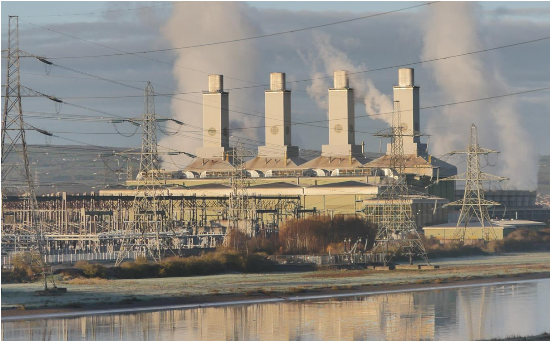
Plate NTS 10: Existing Connah's Quay Power Station (view from Dee Estuary)
